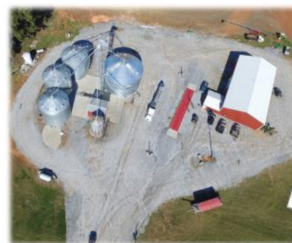
Aerial of ASR Grain Facilities
