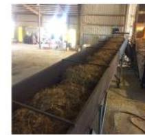
Conveyor system & electrical improvements - $18,000
